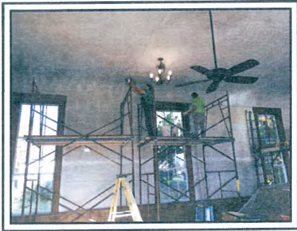
Clockwise from left to right: Sheetrocking in Murray Hall; Painting once the rock is up; A skilled team from Sheetrock Inc. works on the ceiling; More craftsmanship as the job is almost complete
